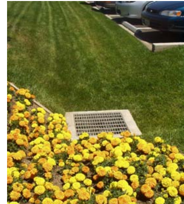
Parking lot drains to vegetated swale, Union City
