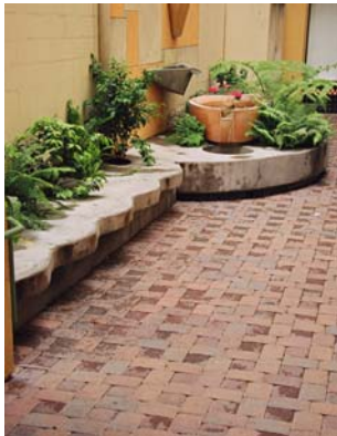
Ungrouted modular pavers promote infiltration, Berkeley
