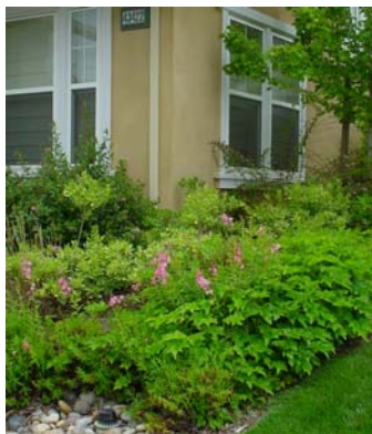
Rooftop runoff drains to bubbler in landscaped area, Fremont
